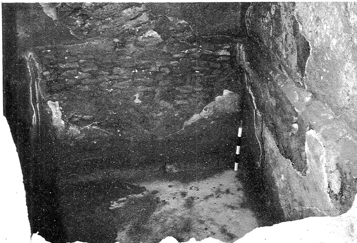
1 Inside of water reservoir
