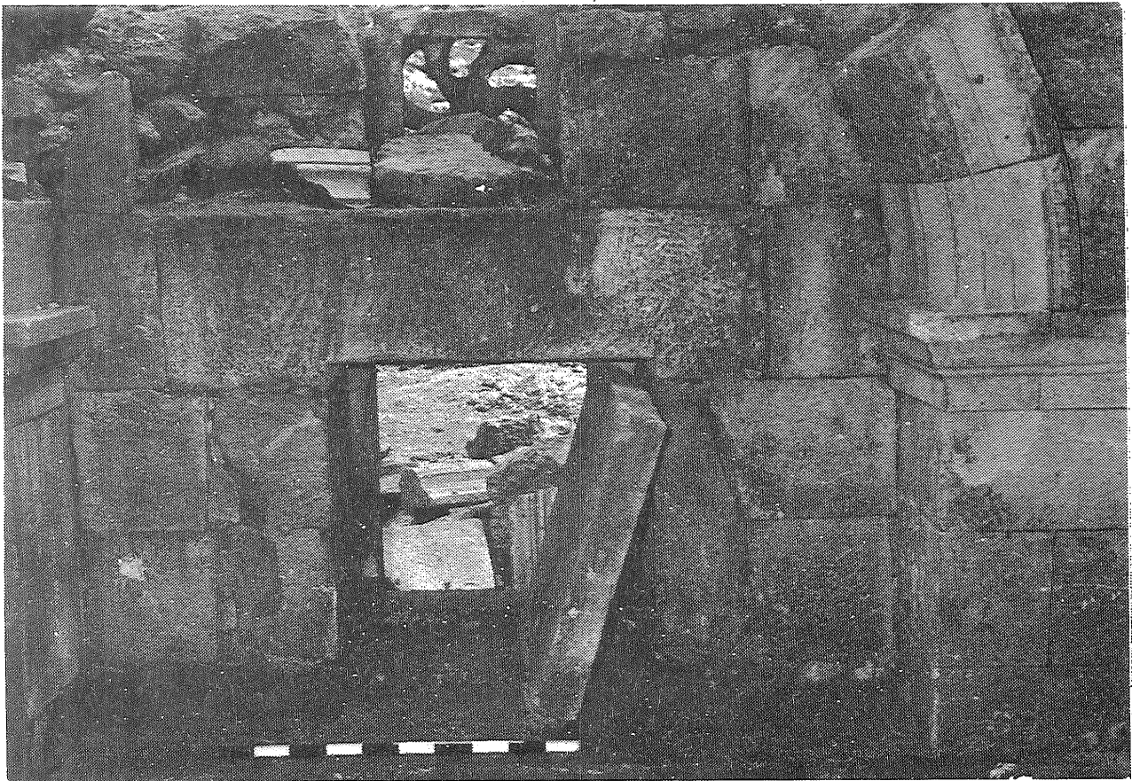
2 Doorway after clearance seen from inside
