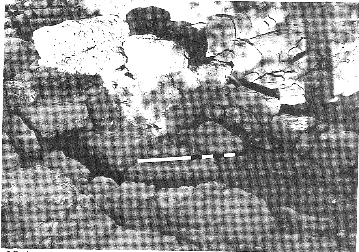
2.D. Area : Extended drain in fortification wall, and drain of House Phase 2.
