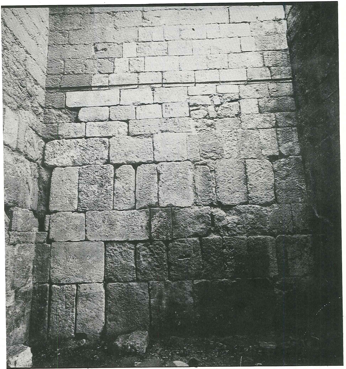
Fig. 4: The west wall of the northeast room after the restoration.
