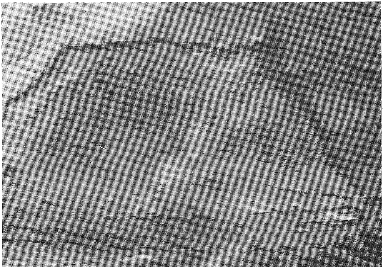
Pl. XL: 2: Erosion at southeast corner of site; looking northwest.
