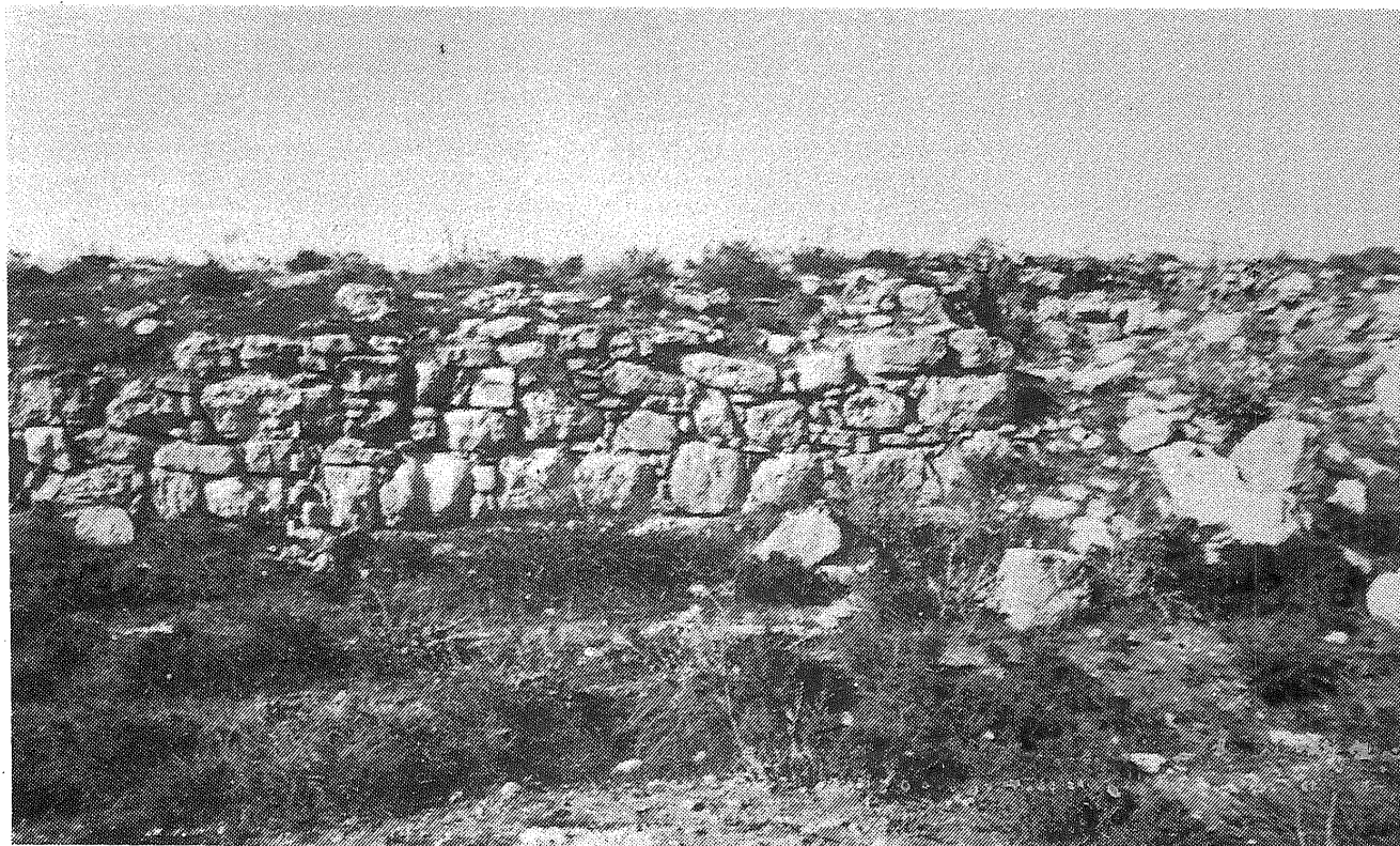
Pl. LVI: 1: Construction of installation wall at Khirbet Salameh
