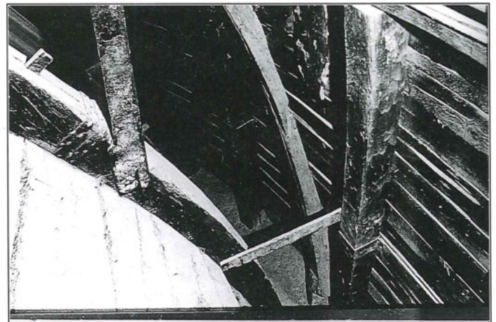
18. Al-Aqşa mosque. Beams of inner dome and scarfing technique.
