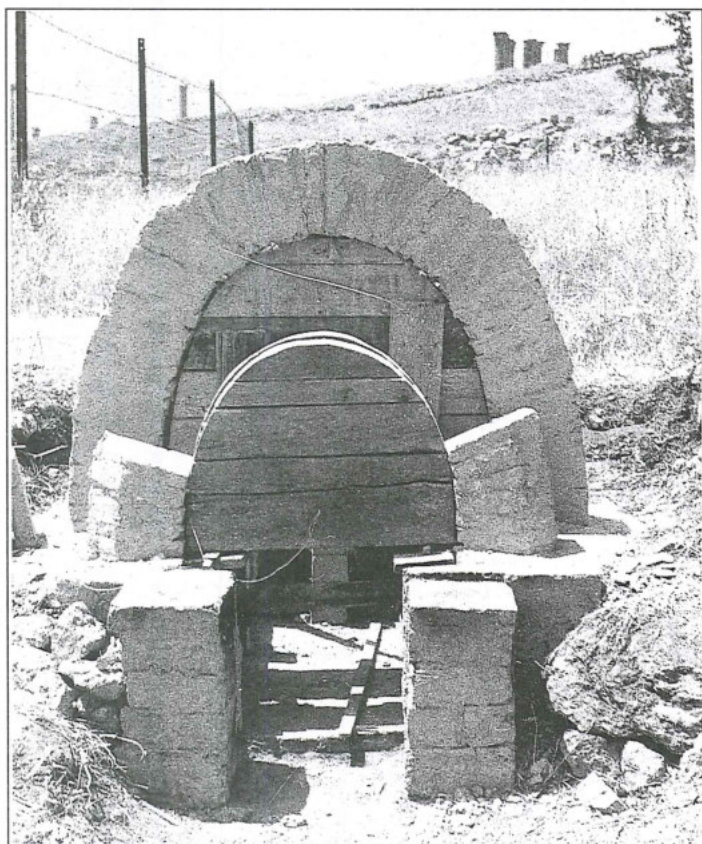
4. Building the superstructure arches.
