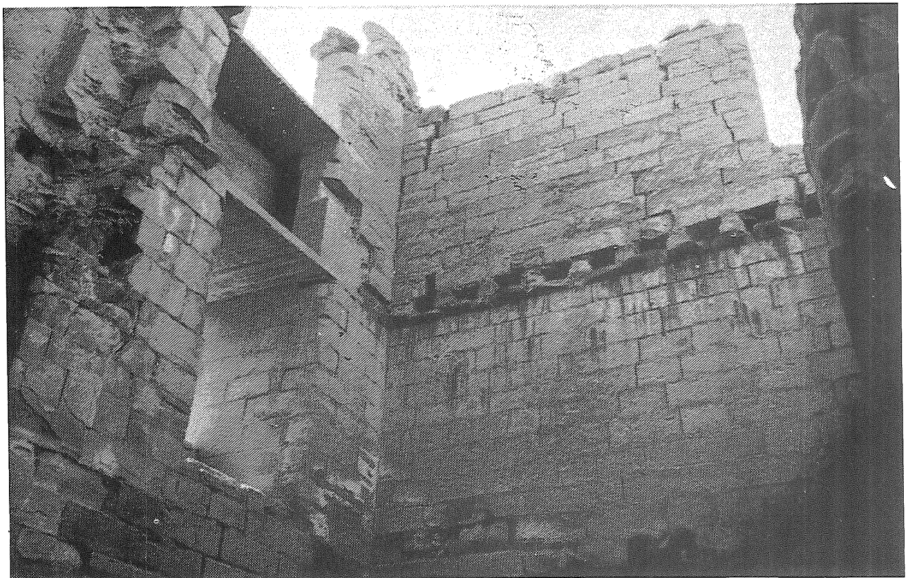
2. Interior of Compartment 1, showing roof-beam emplacements. Looking S-E.
