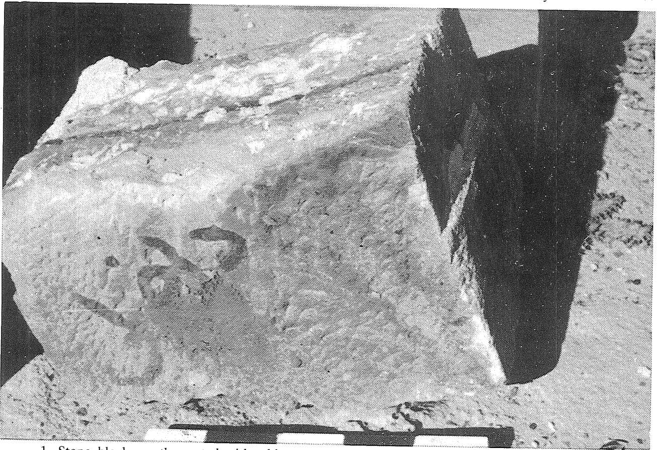
1. Stone block, partly coated with white stucco found in the core of the N-E anta .
