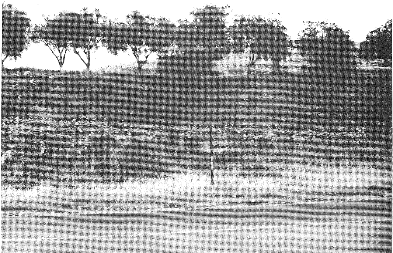
2. General view of the eastern cut of Sweileh-Jerash road- Looking East.
