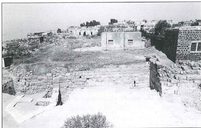
1. Hellenistic city wall with pentagonal tower (photo: R. Wiczorek).
