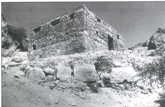
2. Modern bathhouse at Hammāmāt Abū Dhabla, pedestalled above the wādi floor, with earlier Roman-Byzantine wall exposed beneath it (Site 92). View NE.
