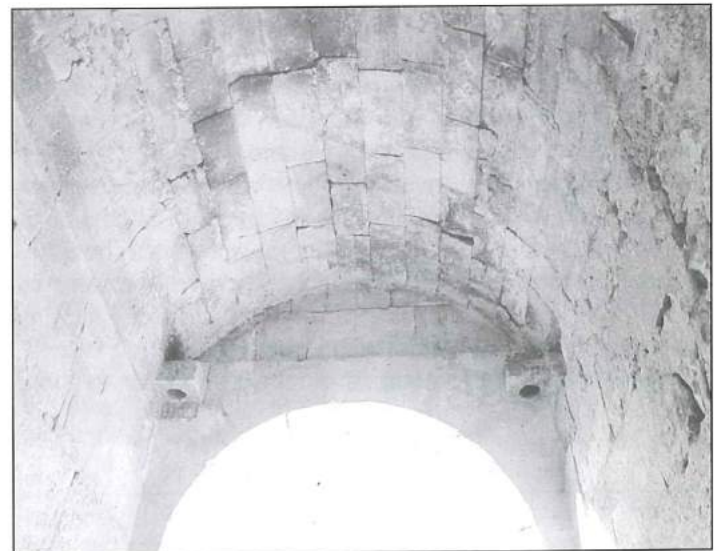
11. Gerasa, Hadriatic arch, detail of the door-hinges in the passage-ways. (Photo by Th. Reiss).
