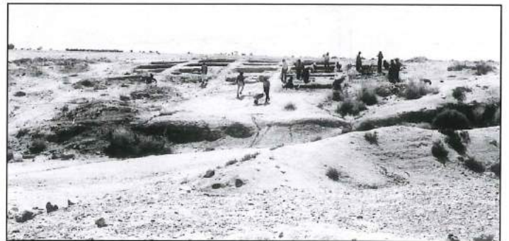
5. Part of the excavated area south of Tall al-Kharrār.
