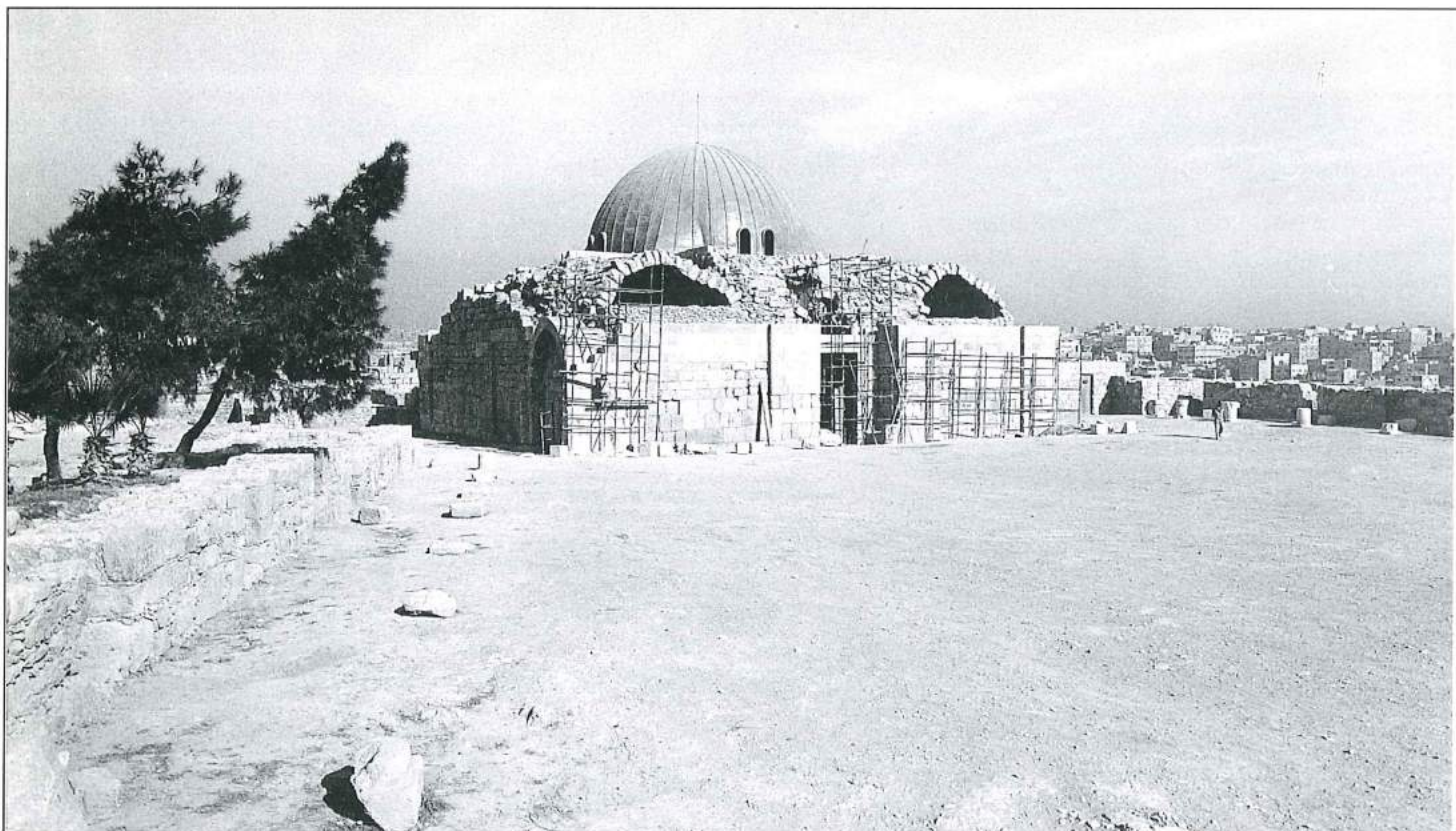
5. The entrance hall from the south.
