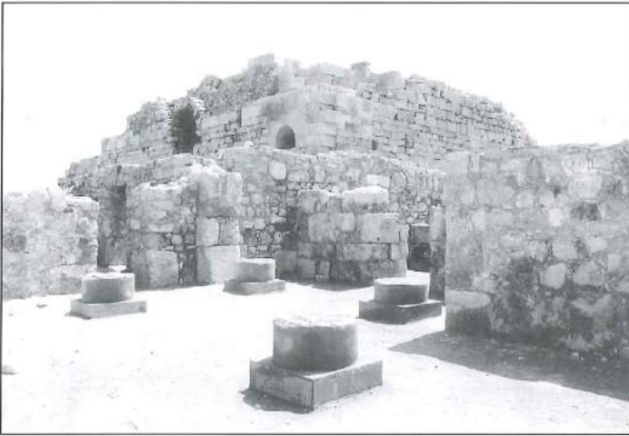
5. The building structure before the dome was built (photo by I. Arce).
