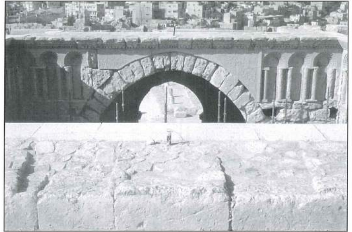
4. View from the top with evidence for sills of two windows.
