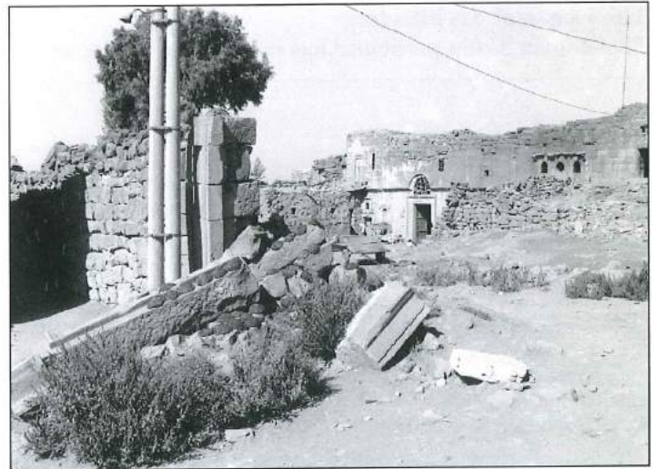
1. Destroyed portal of gateway leading to the compound of the historic mansion at Inkhil, Syria (photo: F. Aalund, 1988).
