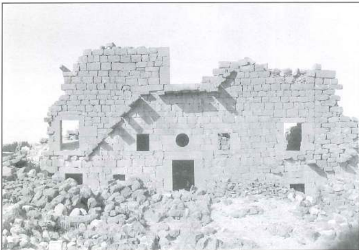
3. Two storied main facade with corbelled staircase to second floor. Umm al-Jimāl, Jordan (Photo: F. Aalund 1985).
