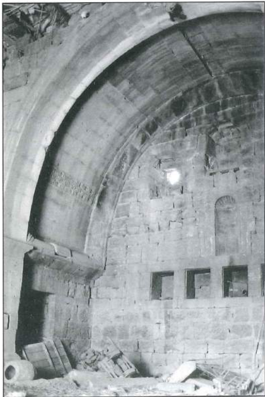
10. Large stone vault in ovoid shape at the rear of the mail hall, mansion at Inkhil, Syria (Photo by F. Aalund, 1988).
