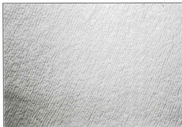
18. Diagonal dressing of the stone.
