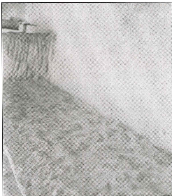
16. Tool marks on top of pediment.
