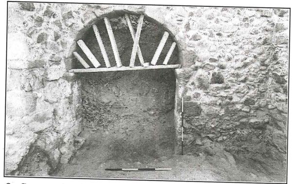
9. Supporting arch under north aisle of church, F. I 4.1/H. II 7 (Photo T. Springett).
