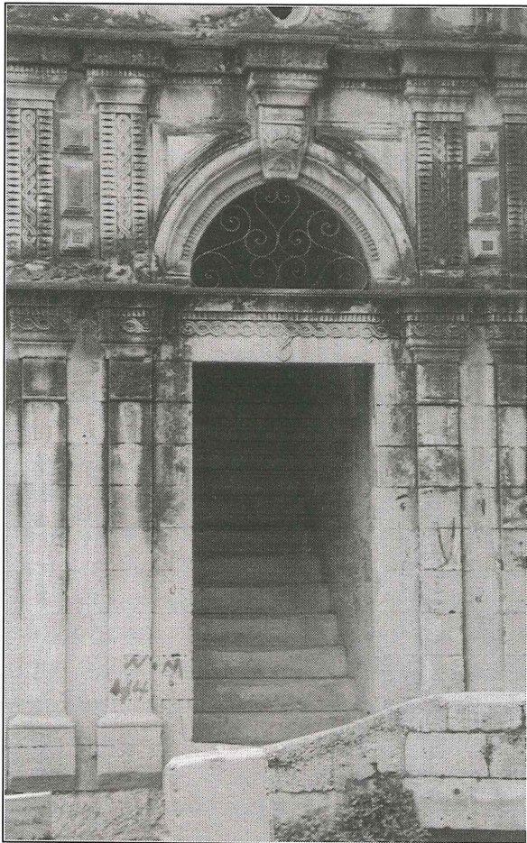
8. Main portal of the Bayt Abujaber.
