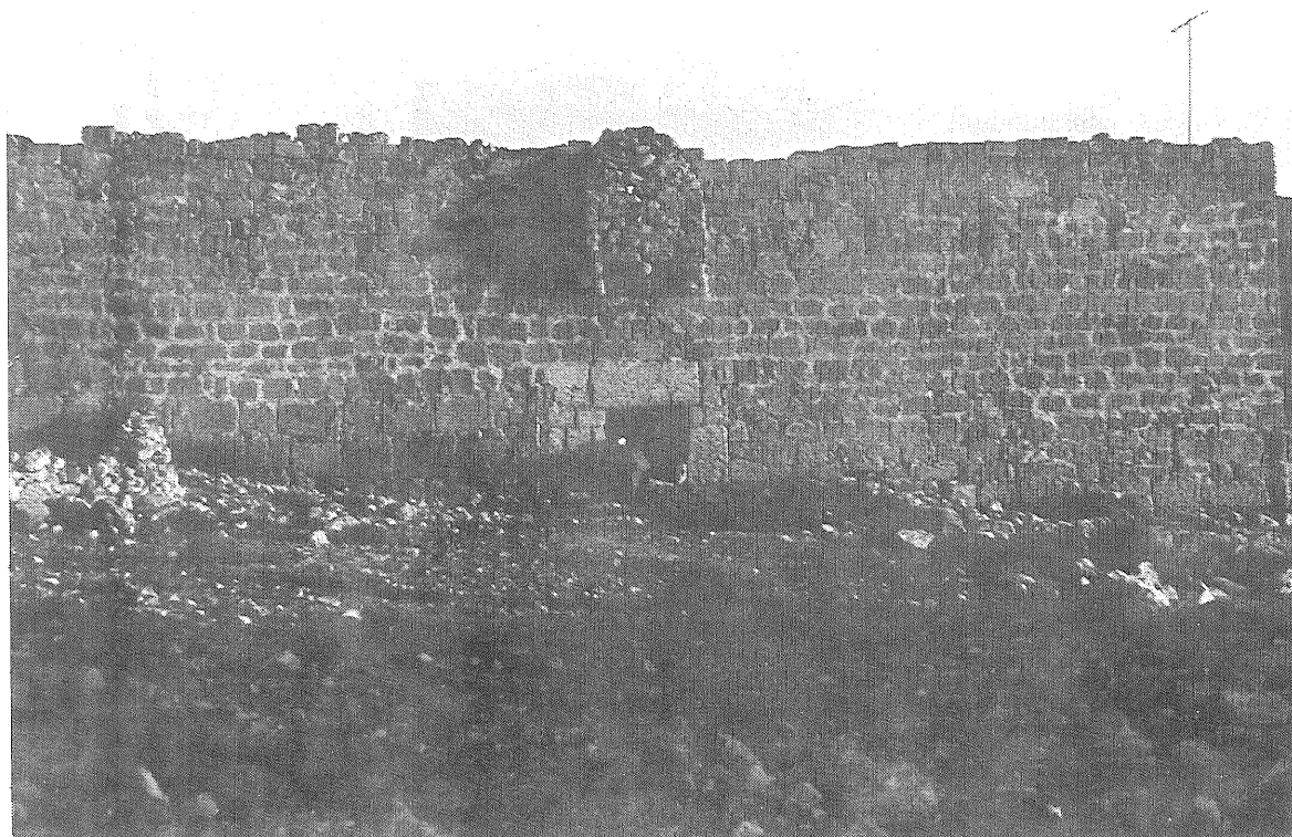
Pl. LII,1: Ottoman fort, main facade, looking north.
