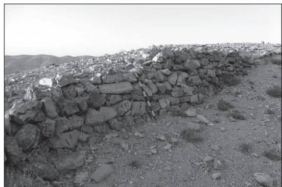
8. Retaining wall of the reservoir at Boz al-Mushelle, looking north.
