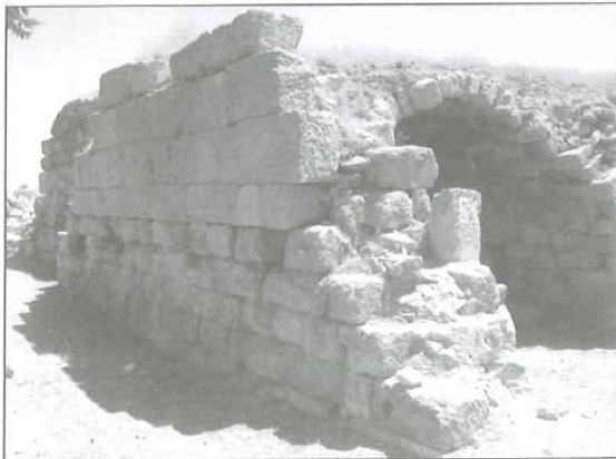
2. Qasṭal al-Balqā'. Umayyad wall from the 'Syrian bayt ' to the north of the entrance block/vestibule (facing the court corridor), which presents two different building techniques corresponding to two consecutive building phases (both datable to the Umayyad period). The vault seen to the right, dates from Ayyubid-Mamluk period; it is built within the width of the Umayyad room, and rests on its own walls which double the Umayyad ones (see FIG. 3).
