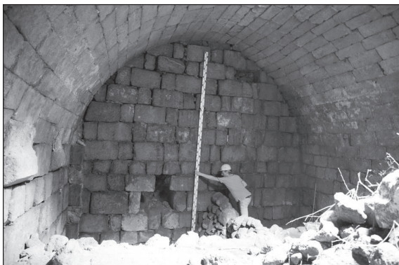
2. Vaulted substructure/cistern in Area III.
