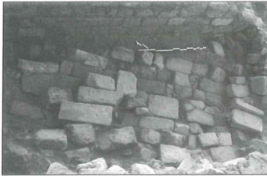
9. Fallen masonry, still closely aligned, within Room B.2, probably the result of the 363AD earthquake.
