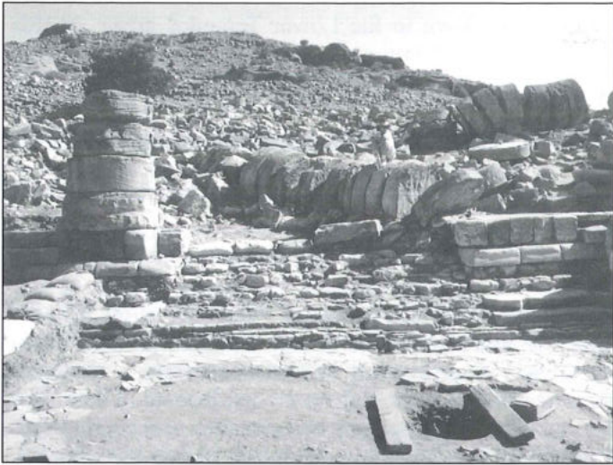
2. Petra Southern Temple Forecourt, showing the area of disturbance in the foreground, 1994, facing south.
