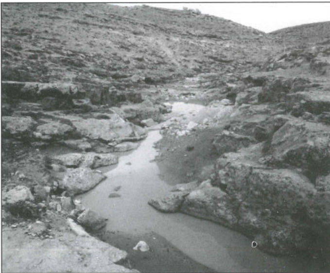
18. Remnants of dam lake infill in the upper reaches of Wādi al-Lāhūn.
