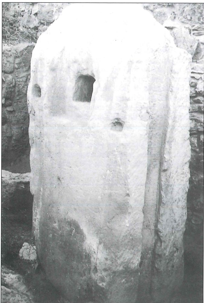
7b. Right pier with unlevelled two notches to hold the weight rod.
