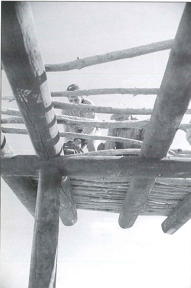
27. Branches Being Laid in Place.
