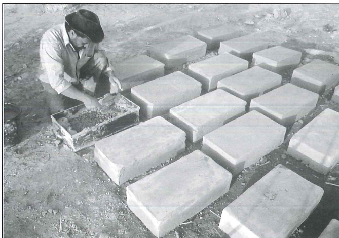
30. Fashioning of Concrete Mudbricks.
