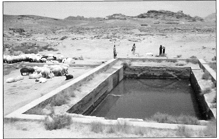
3. Reservoir in settlement centre (survey nos. 67), view.
