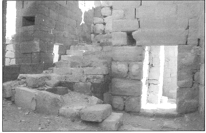
6. Tower 22. Detail showing the rusticated corner ashlars from the first quadriburgium tower comprised in the second quadriburgium one.
