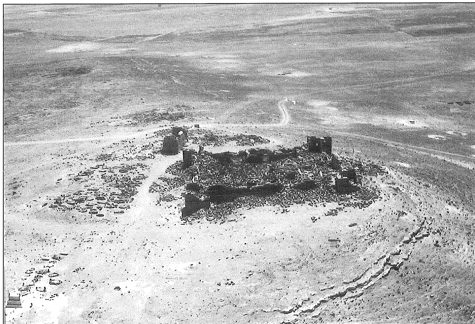
2. Aerial view before the intervention.
