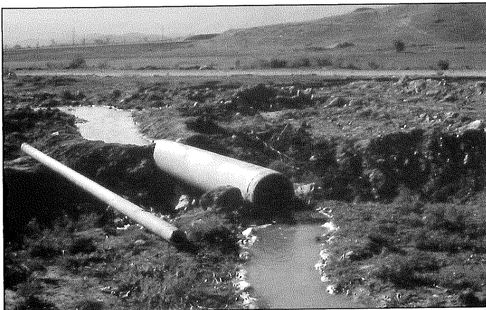
2. Temporary irrigation channel dug in the Ghawr ar-Rāma, north-east of Tall Iktānū, a concrete pipe has been used to bridge an army excavation. IKS643; photograph Kay Prag, January 1989.
