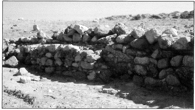
6. The east wall of the tank at Muhtariqa, with steps at the north-east corner; from the south-west. IKS1243; photograph Kay Prag, 27/9/95.
