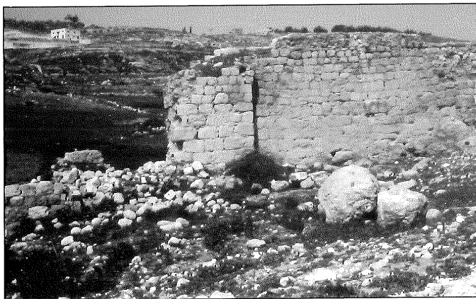
4. Water mill in the Wādī Ḥisbān, just south of Shunat Saqr (Ibach 1987: 226; Prag 1991: 50, fig. 3, incorrectly identified as the barn of Diyab). The aqueduct/leat is on the right, the drop shaft on the left. The mills were repaired at various times, and the masonry in this mill is testimony to three or four phases. There are quite large, rectangular, dressed (probably re-used Roman/Byzantine) masonry blocks visible in the lower four courses, at least one phase of smaller, squared blocks above (Ottoman period?) with rubble exposed at the top. HIS10; photograph Kay Prag, spring 1992.
