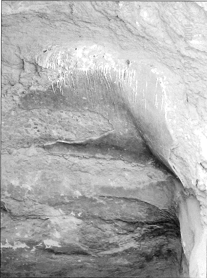
14. Detail of the plastered wall of the cistern.
