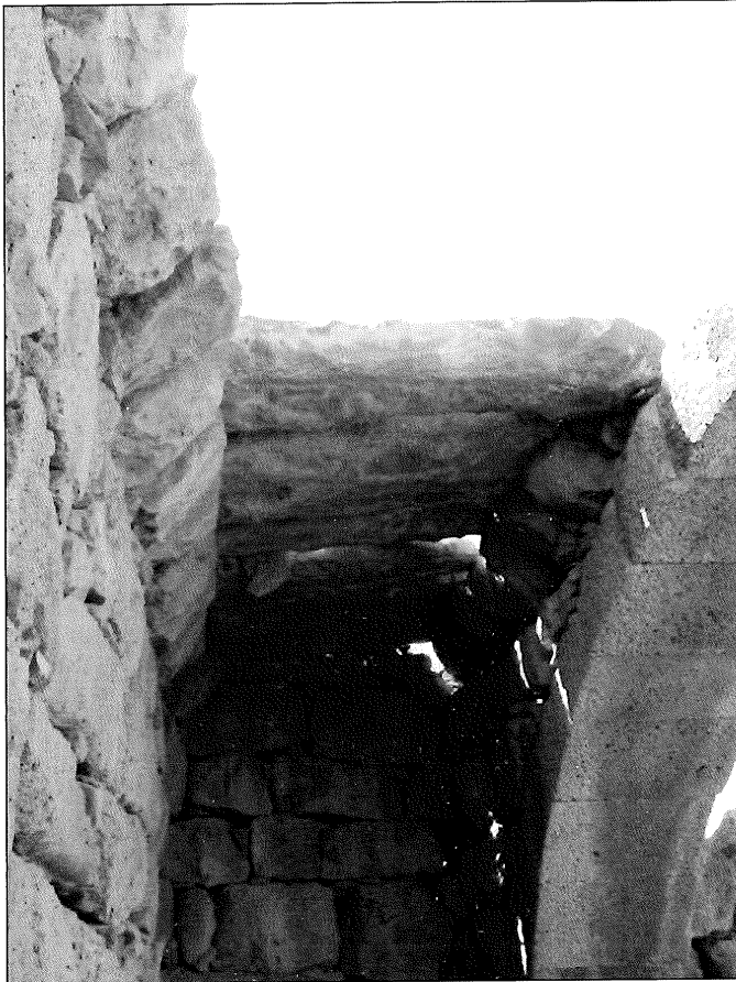
10. Roofing with a large blocks.
