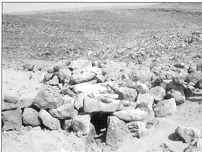
8. The dam after restoration.
