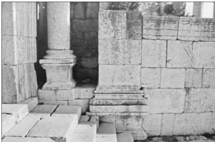
8. Detail showing the relationship between the column pedestal of the monumental doorway and the second-century pilaster (WB).
