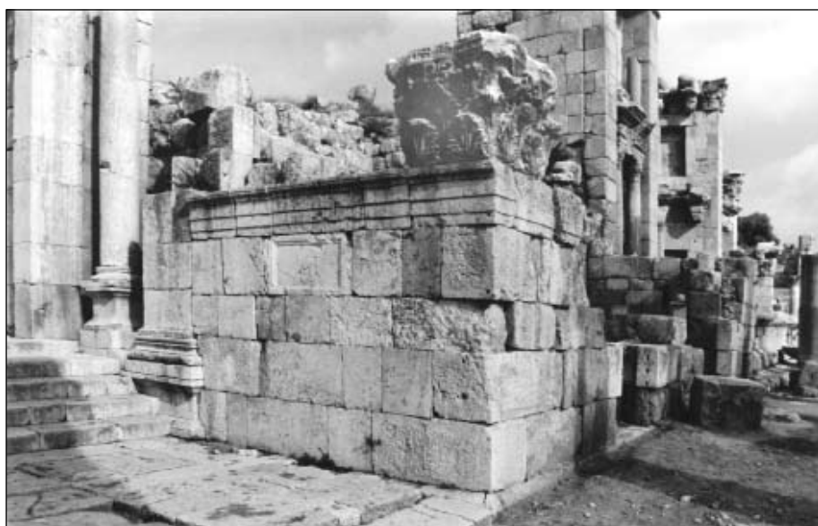
5. North side of propylaeum with the nymphaeum visible in the background. The second century pilaster can be seen on the left, clearly abutted by the Late Antique structure in the centre of the picture. The pilaster capital now sits on the corner of the later structure (WB).
