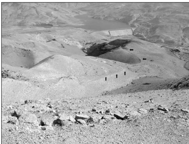
5. The wide sections of Naqab Arar as seen from the upper part of the naqab .
