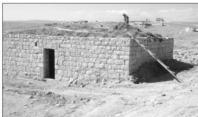
14. Folklore Museum during restoration works.
