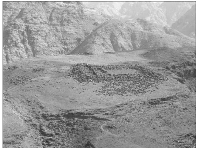
10. An overview of Rās al-Miyāh East, looking towards southeast. The fortress is located on the dark Burj formation plateau and built almost entirely of bright sandstone. Note some of the small structures and the arrangement of building stones in front of the northwestern wall of the fortress. The size of this fortress is indicated by the two people standing along the southern corner of the structure.
