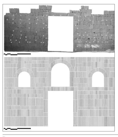
5. Hallābāt room 24 (reception hall). A: Mapping the holes drilled / carved on the basalt-built northern wall to take the metal cramps which held the marble slabs that lined this reception hall in place. Note, at floor level, traces of the thick (2 to 4cm.) mortar layer used to fix the slabs and even traces of the marble slabs themselves. B: Reconstruction of the marble panelling according to the material evidence, *viz.* (cramp holes and imprints of the slabs on the fixing mortar).
