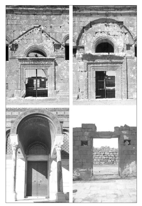
8. Canopies. A and B: Qalb Lozeh church, Syria: traces of two canopies with gable and semi-circular profiles respectively. C: Jerusalem, Dome of the Rock: canopy. D: Hallābāt: traces of a canopy at the entrance to hall 24; note traces of mortar from the vault and holes for the supporting beams.
