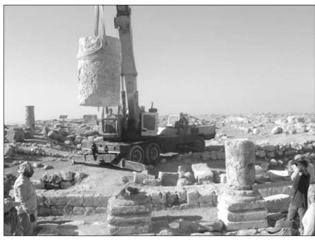
was drilled in the centre of each drum in which to insert the titanium bar. Additionally, a lead sheet (2mm thick) was set on the base of each column to improve levelling.
