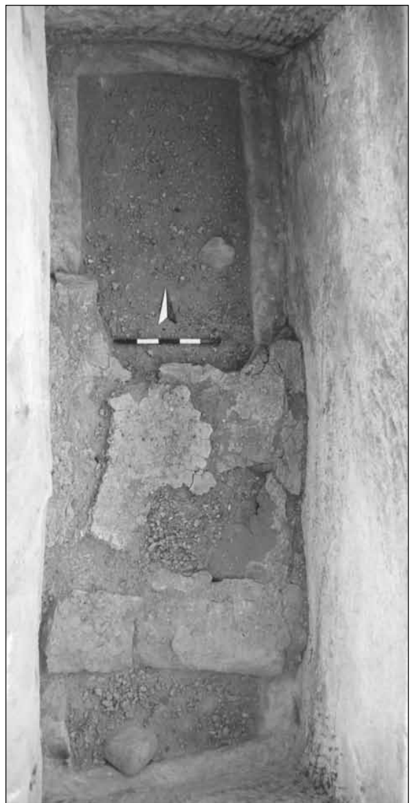
12. BD 24. Broken covering slabs and mortar in loculus ST1 (L. Gorgerat).
