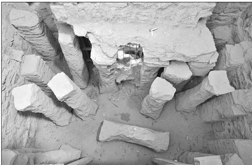
3. Scattered pilae in the caldarium before intervention.
