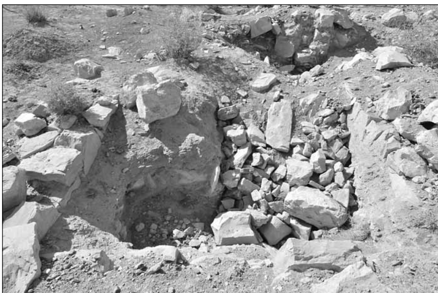
14. Poor state of conservation of the second saqiya .
