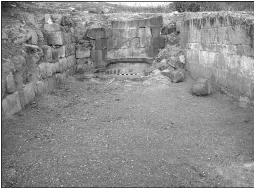
3. Basalt installation from the west (photo courtesy of the British Museum).
