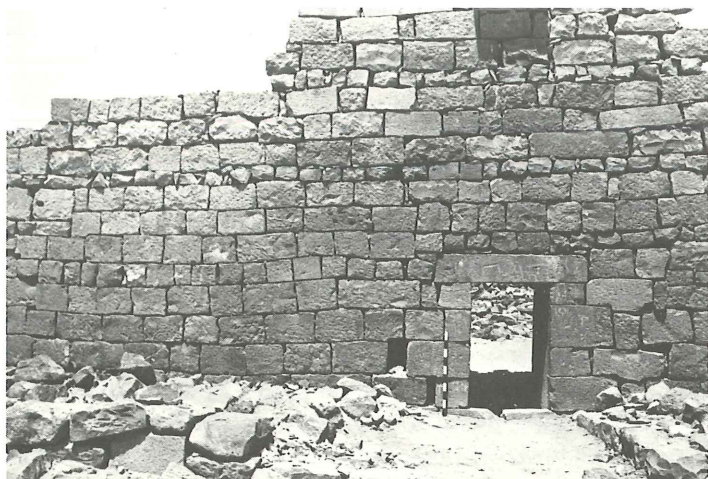
3. Facade of Barracks showing rows of corbels (from their rear) functioning as cross ties: the fourth and eighth courses above the lintels.
