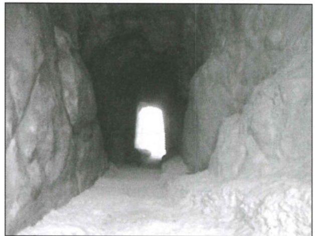
25. Tunnel entrance after clearance of rock fall.
