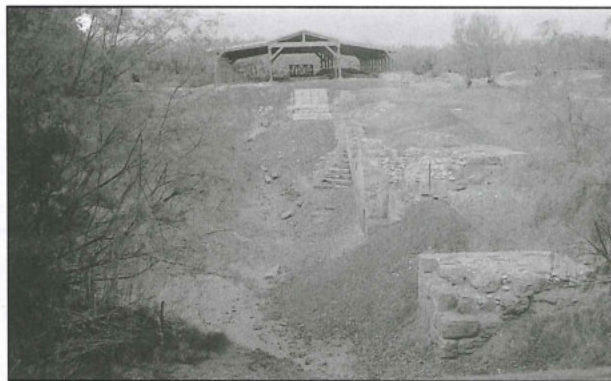
1. The remains of the four piers (Cruciform Baptistery), staircase and basilica (from the east).
