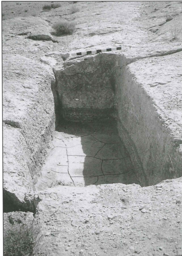
6. This reservoir at Site 490 collects water running down the slope above it.
