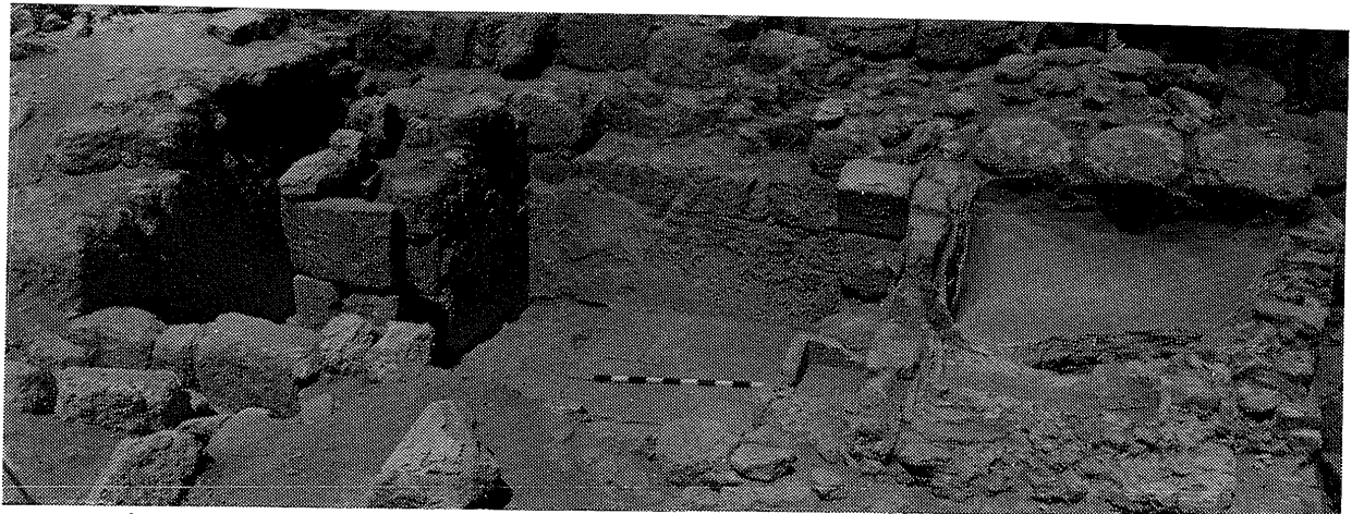
2. The northern half of the Area A Mamluk bath complex. From left: access hallway, bathroom proper with tiled floor and basin, plastered reservoirs, furnace room (P. Bergsma).
