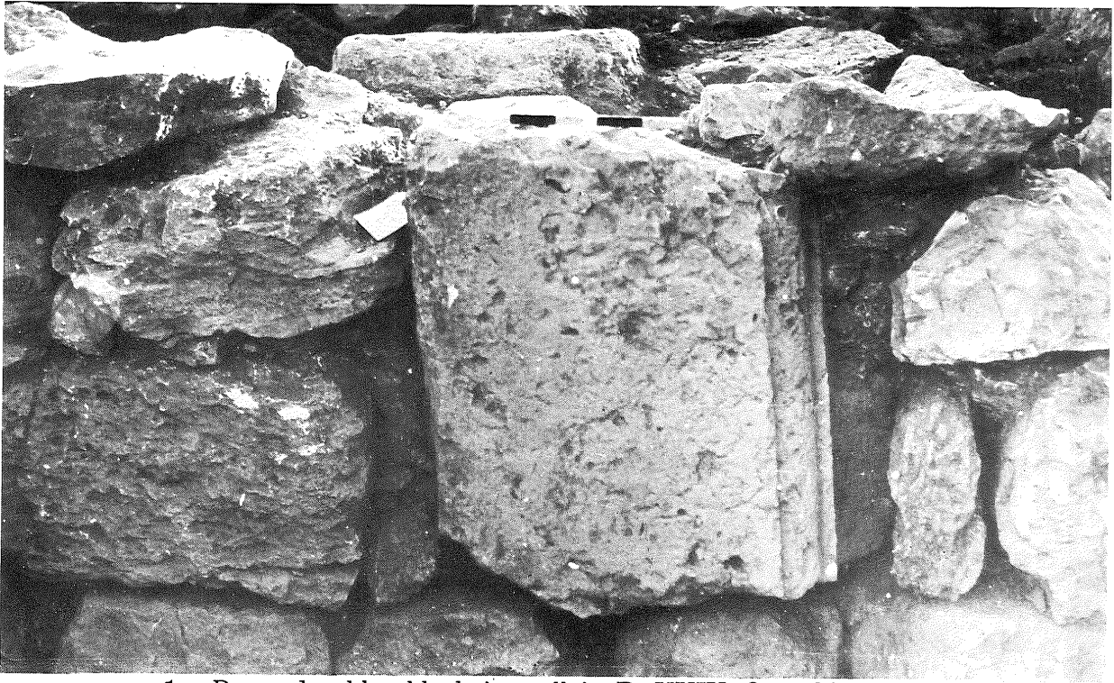
1. Re-used ashlar block in wall in B. XXIV. 2. looking east.
