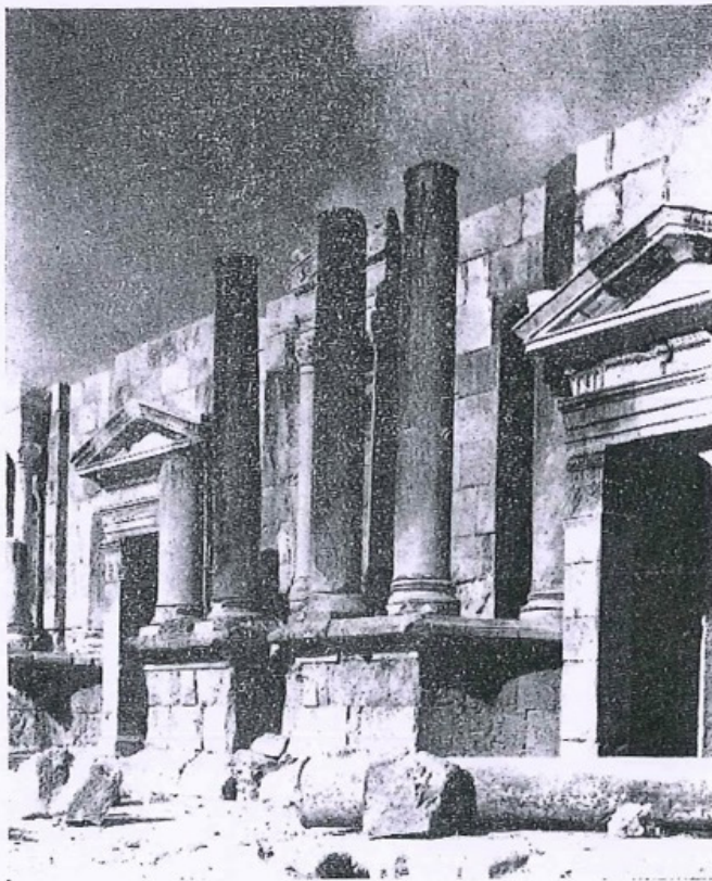
2. JERASH- THE RESTORED EAST AND CENTRAL DOORS AND EAST CENTRAL NICHE.
