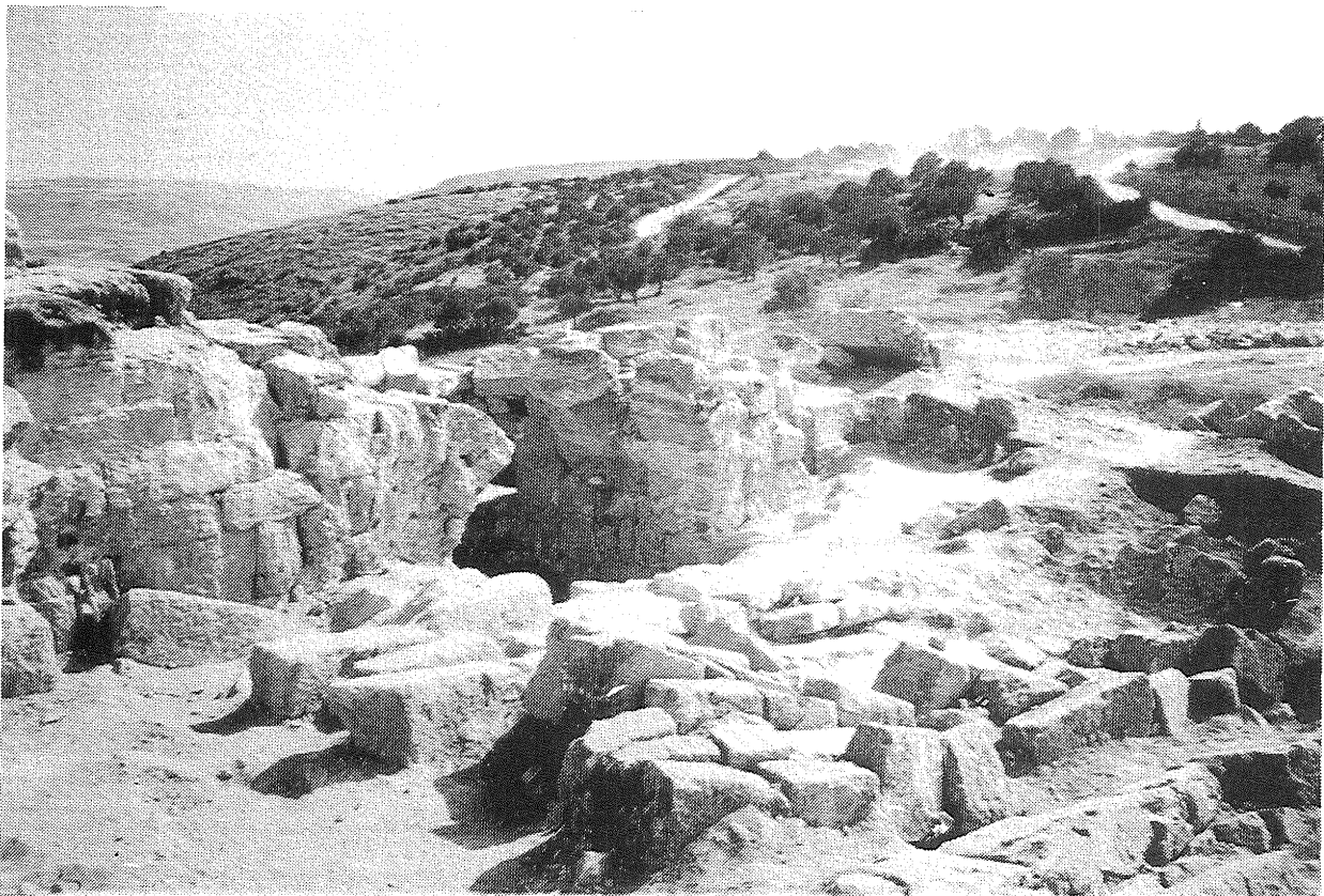
2: The fallen barrel vault of room III.
