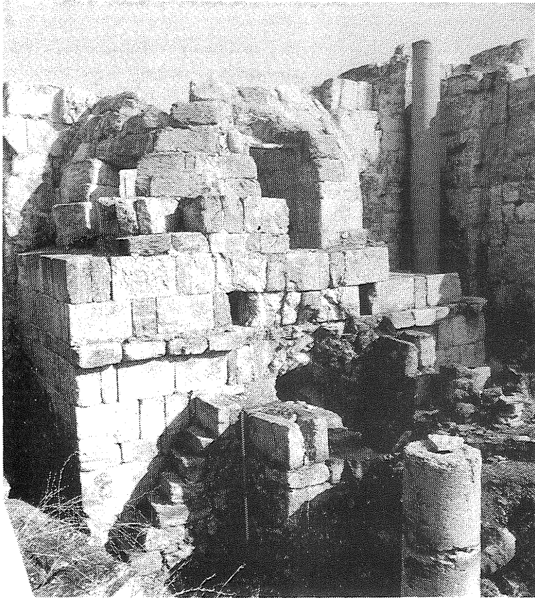
1: Room I, apse II, built up against the north wall of the room in the second Bath Period, seen towards the northeast.
