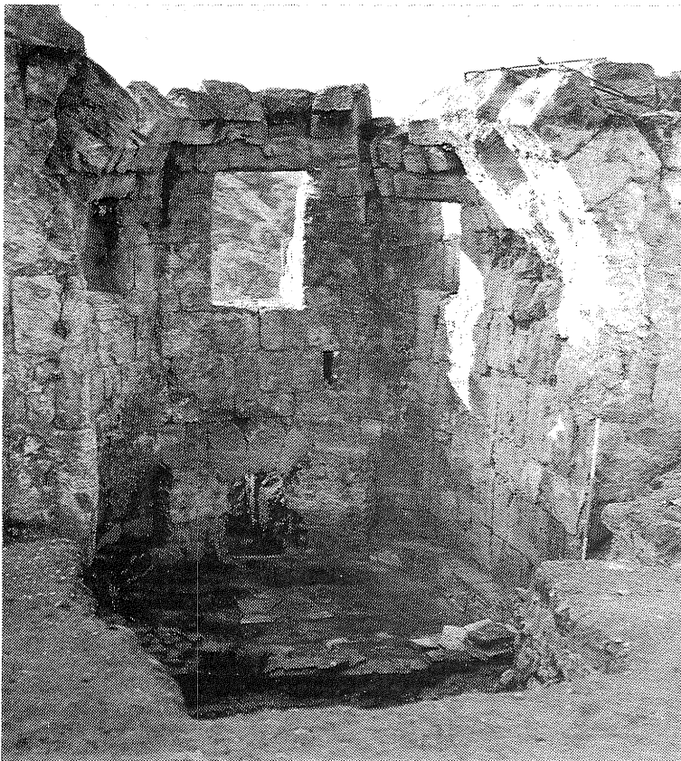
2: Room III, the apse II with the hot bath ( alveus ) seen towards the south.
