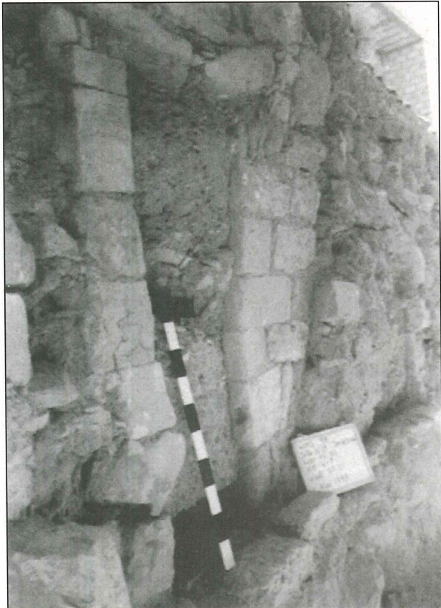
17. Completely preserved doorway connecting two rooms in a Nabataean villa at Dār al-Birka (W18).
