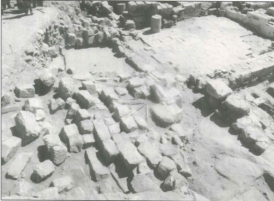
3. EZ IV. Main entrance, Courtyard 28 and collapsed façade, seen from the northwest (photo D. Keller).
