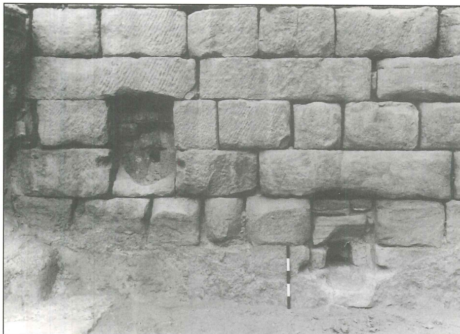
19. Retaining wall of cistern on the upper terrace with two water spouts (photo Schmid).
