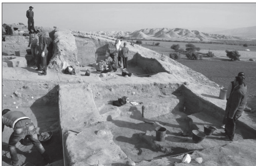
1. Excavation work in 2014.
