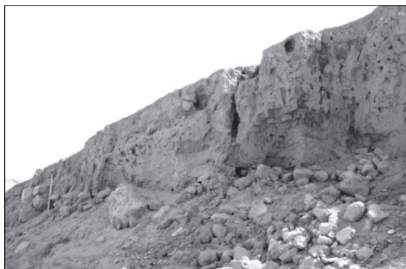
18. Tall Blaibil: remains of mudbrick fortification wall (Photo: A. Ahrens).
